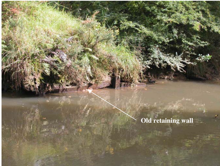
Figure 4 Old retaining wall on Reach 8 Ch450
